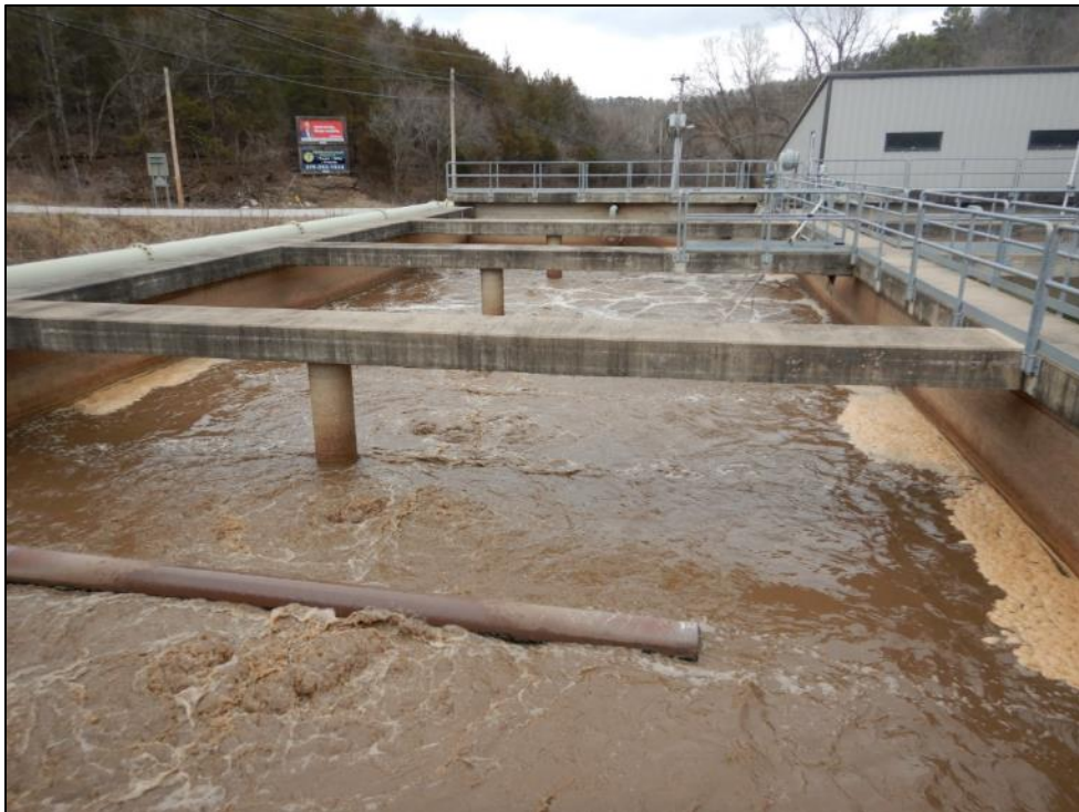
Photograph 6. The western SBR basin during the react mode.
