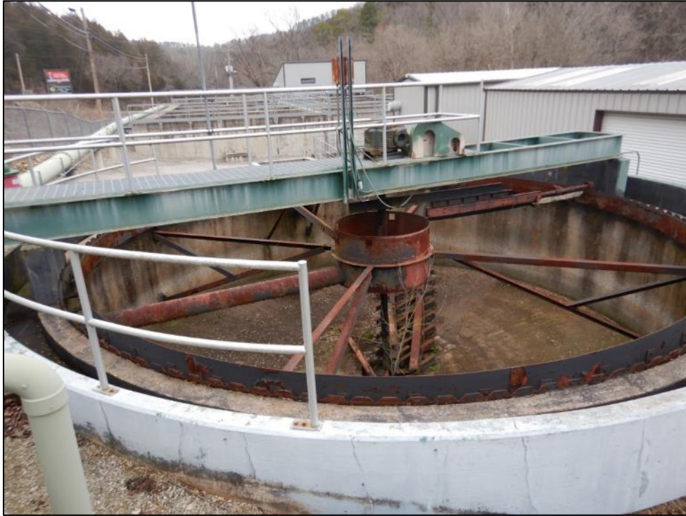
Photograph 5. Decommissioned clarifier that could be used for wet-weather storage.
