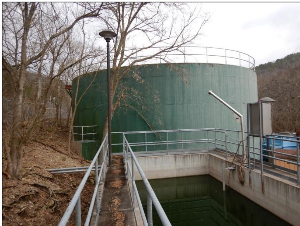
Photograph 12. Decommissioned trickling filter that could be used for wet-weather storage.
